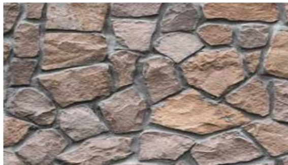
Figure 1.1 Rubble masonry wall
