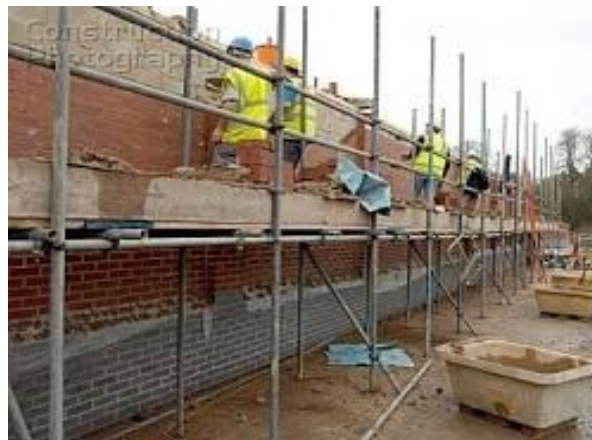
Figure 6.13. Single scaffolding
