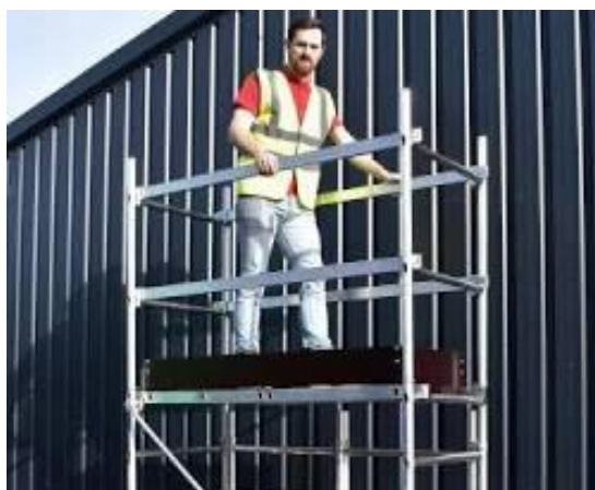
Figure 6.17. Tower scaffolding
