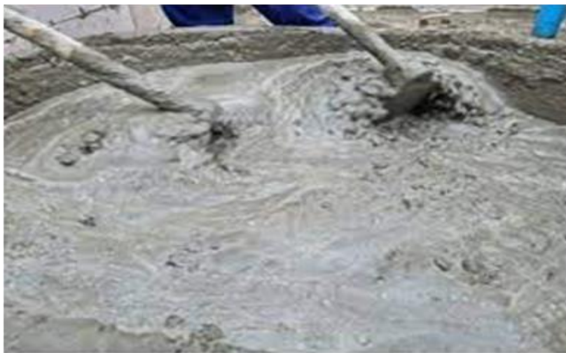
Figure 4.5. Wet Mixing
