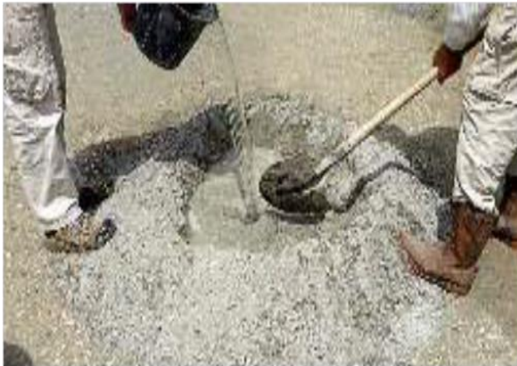
Figure 4.3. Adding water to the dry mix
