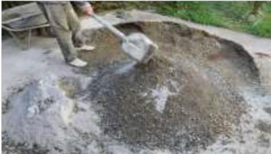
Figure 4.2. Dry mixing
