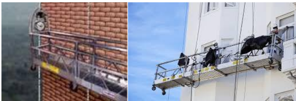
Figure 6.19. Swinging scaffolds
